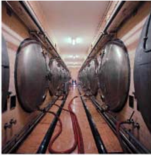
Stainless steel tanks for beer storage
