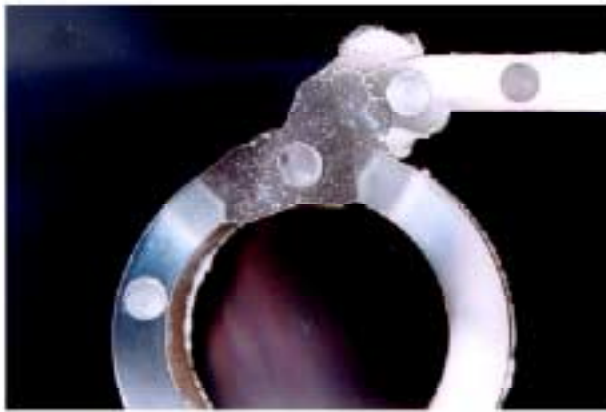
Cracked weld in stainless steel
